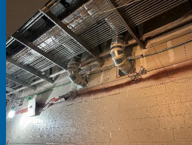
Installation of round pipe and fire dampers in Area C
