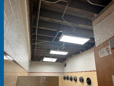
Demolition of hard ceiling in restroom of Area D (East)
