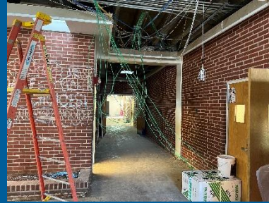
Intercom and Burglar alarm wiring installation in Area E
