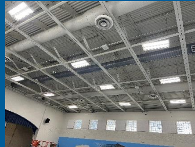
Installation of spiral duct in Area A
