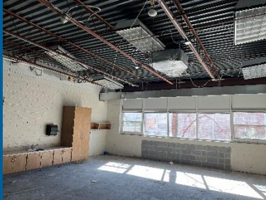
Installation of duct and fire smoke dampers in Area D (West)
