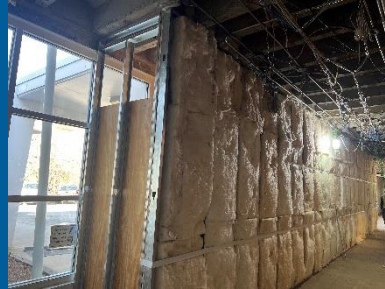
Installation of temporary partition at main entrance to building
